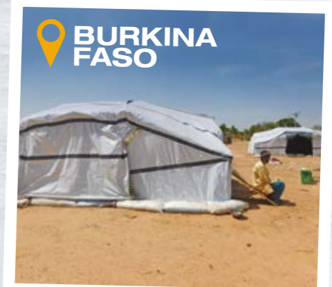
BURKINA FASO Thousands of people fleeing violence now live in displacement camps in Burkina Faso. These 'Sahelian Tents' utilise tarpaulins stretched over a metal frame, with large door openings for cross ventilation.
