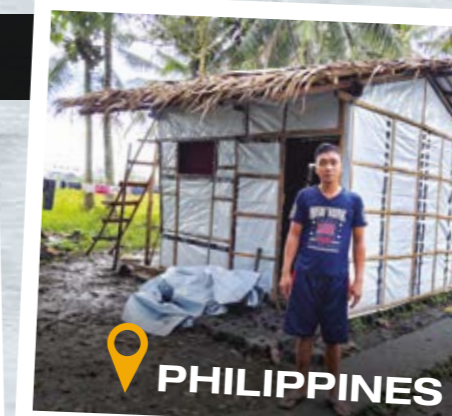
PHILIPPINES Following Cyclone Trami, people needed to construct temporary shelters before the next storm arrived. Here, the tarpaulins are held in place by batons over a bamboo frame and used to make the roof watertight, under a layer of palm leaves.
