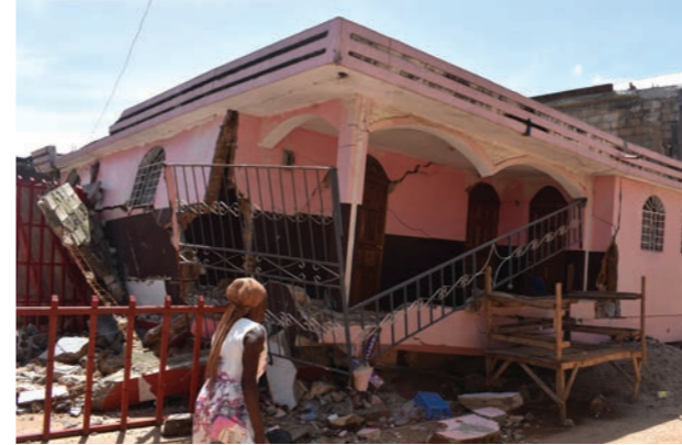
Damage caused by the earthquake in Haiti, 2021. Habitat for Humanity
